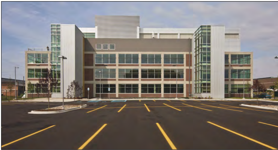
These before and after photographs clearly show the dramatic transformation of the former Franklin furniture warehouse into a vibrant urban school.
