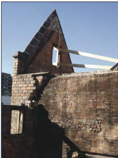
The Monahan Company disassembled, reframed and resupported the roof. The firm also preserved the original masonry, including the gables and chimneys.
