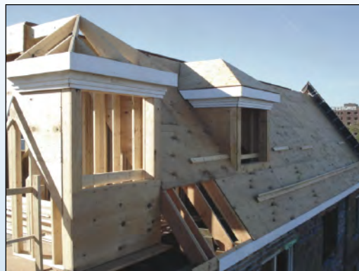
The Monahan Company disassembled, reframed and resupported the roof. The firm also preserved the original masonry, including the gables and chimneys.
