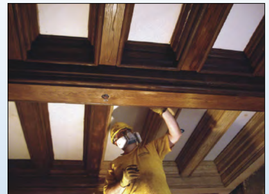
The crew meticulously restored the interior woodwork, including the parlor's coffered ceiling.
